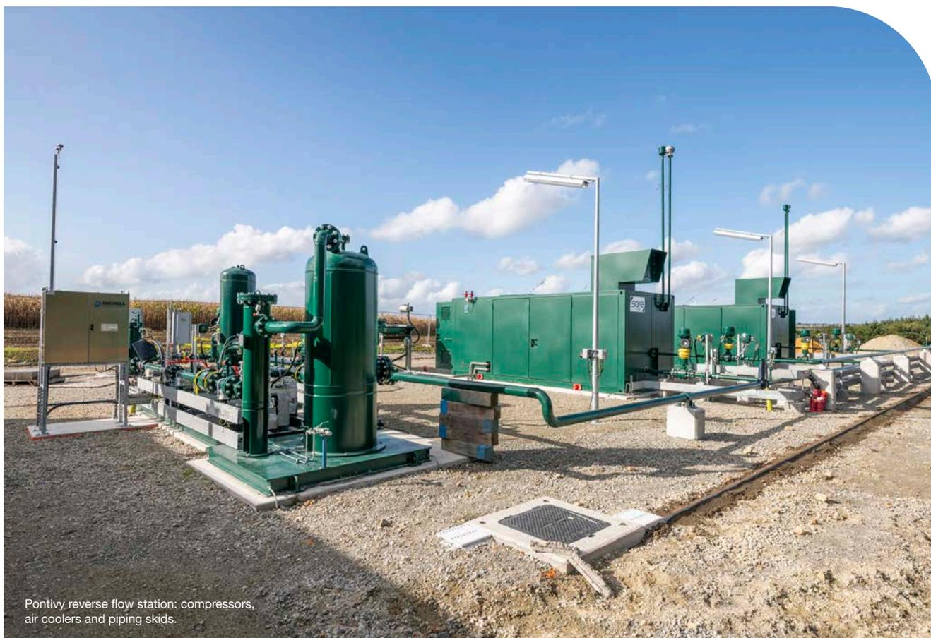
Pontivy reverse flow station: compressors, air coolers and piping skids.
