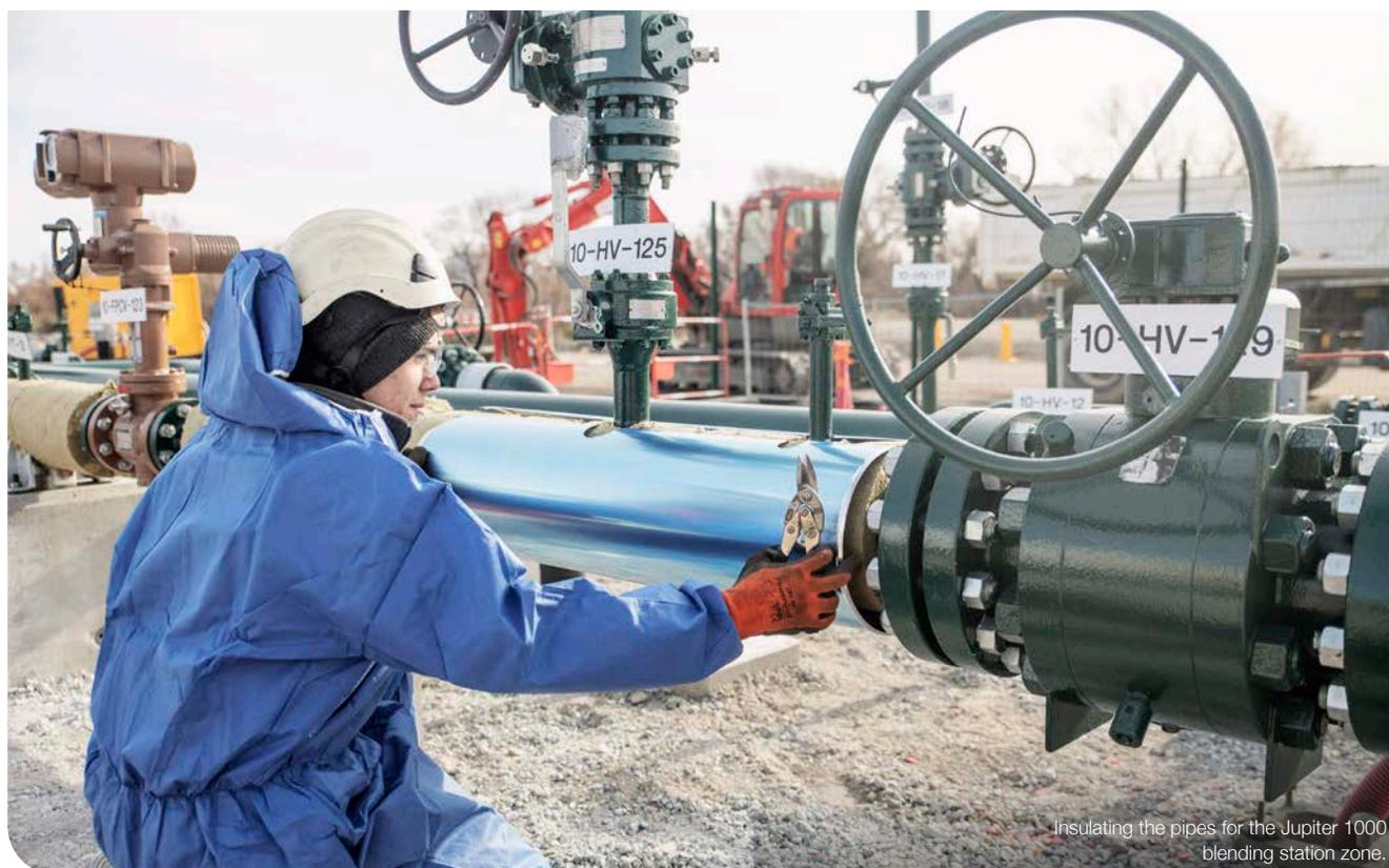
Insulating the pipes for the Jupiter 1000 blending station zone.
